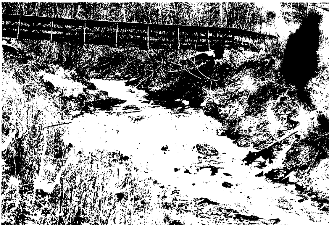
Bridge at Stair Park (Stop 3) before it was washed away, Spring, 1981.
